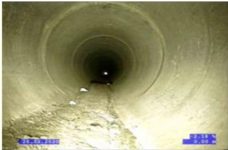
Figure 5 DN1200mm Stormwater Outfall pipe existing condition
